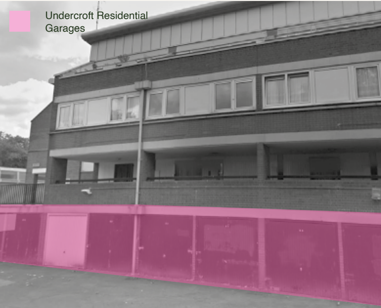
Figure 32: Undercroft Parking Units
