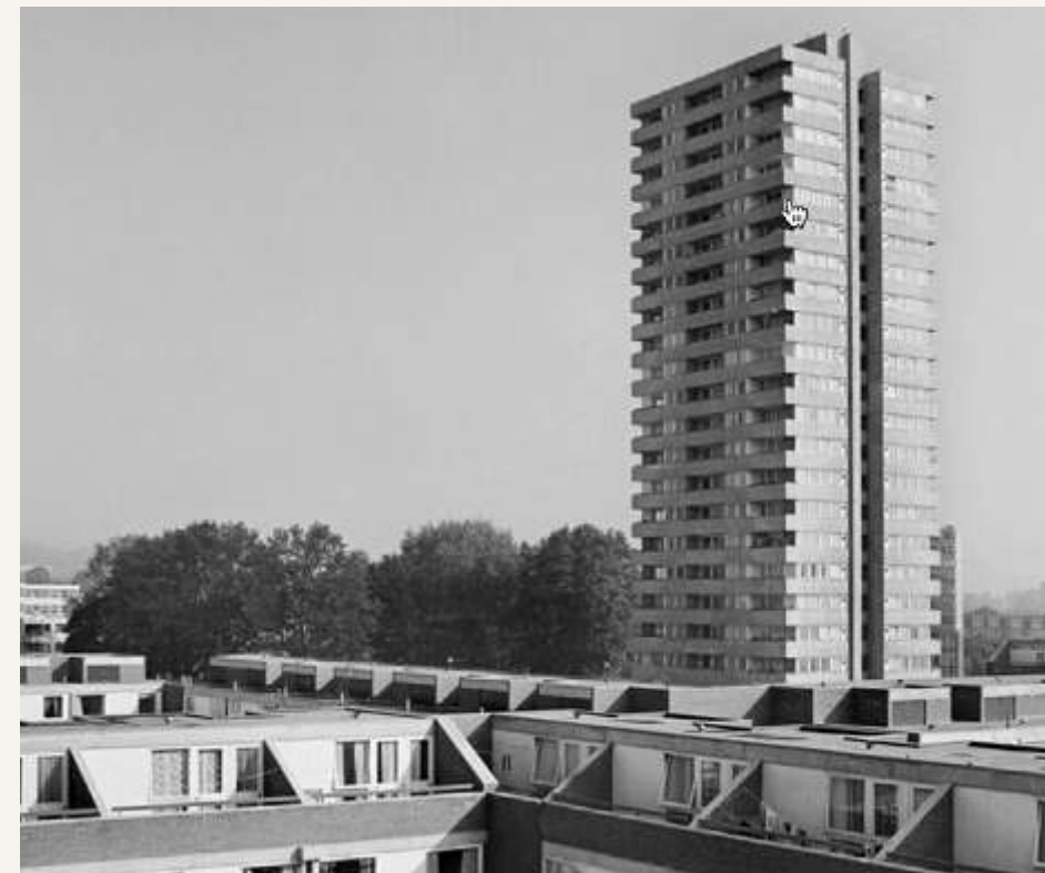
Figure 28: Wendling Estate with Bacton Tower in the distance
